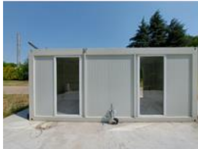
Fig. 3 Container for people accommodation
