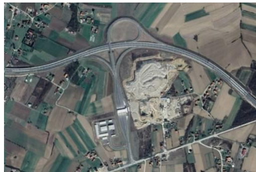
Figure 11b. Highway build up (2018)
