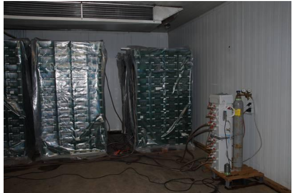
Figure 7. Cherry storage under film caps with controlled atmosphere (CA).
